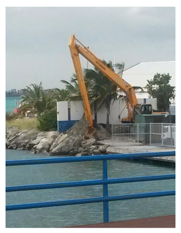
**PHOTO CUTLINE:** Excavator preparing to dredge the section near the dinghy/mega yacht tender dock.
